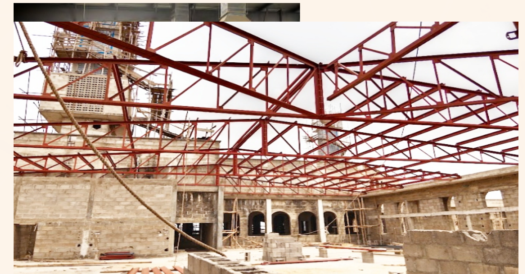
STEEL TRUSS AT NASFAT AGEGE MOWE
